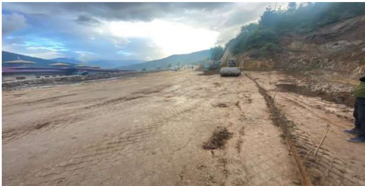
Figure 9 - Ongoing 4-Lane Road Development Project
