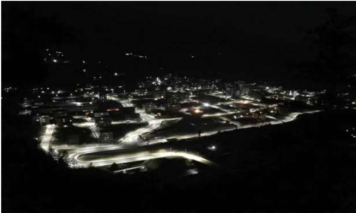
Figure 5- LED Street lighting for Taba LAP
