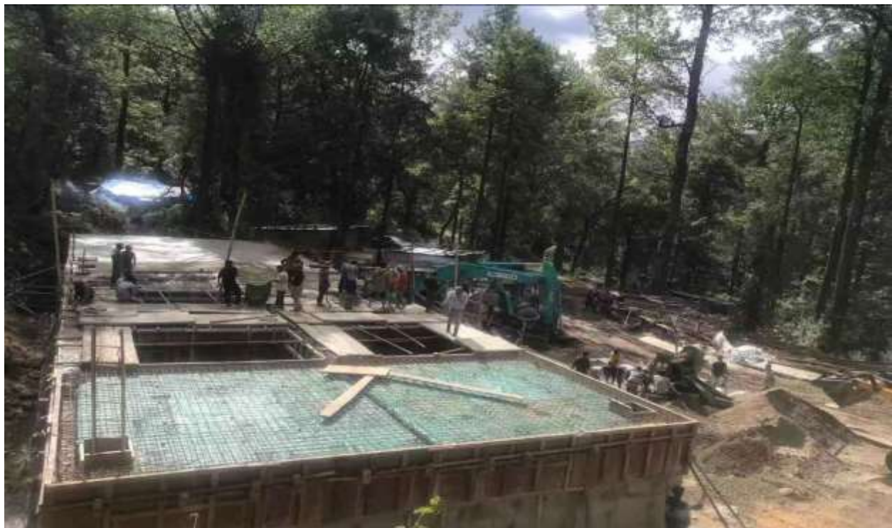
Figure 10 - Ngabiphu WTP (Ongoing)
