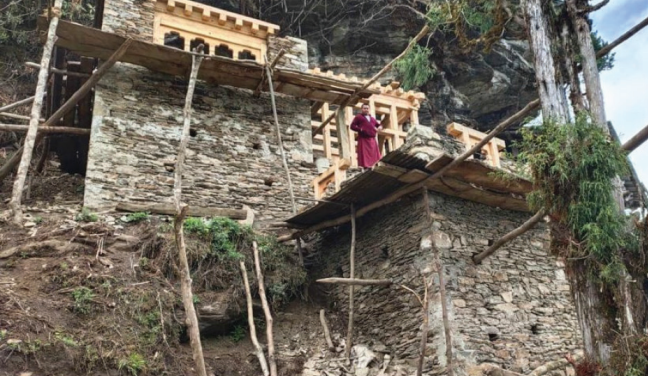
Monitored Construction of Retaining Wall at Dramethang Lhakhang
