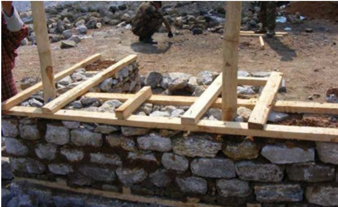
Fig. 20: At Corners and intersections
