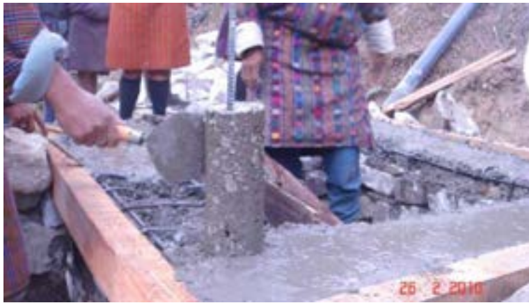
Fig. 33: Steel in Reinforced Concrete Band
