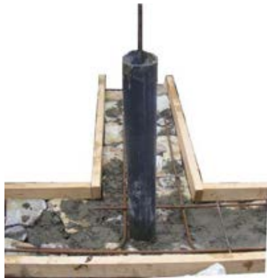
Fig. 33: Steel in Reinforced Concrete Band
