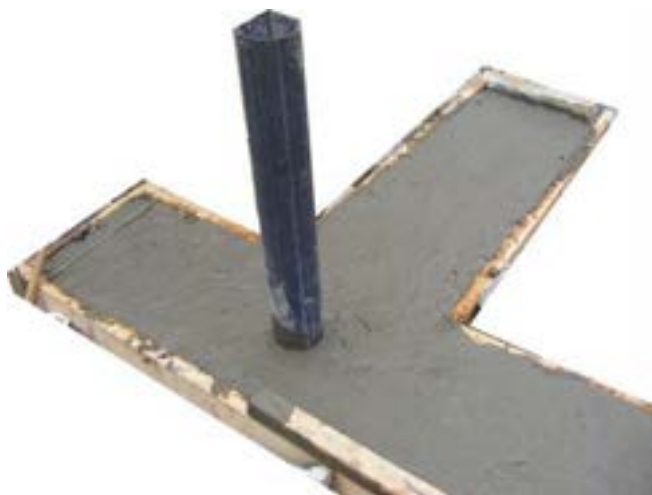
Fig. 34: Reinforced Concrete Band
