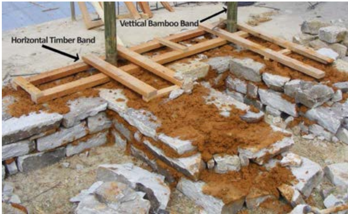
Fig. 15: Vertical and Horizontal Bands
