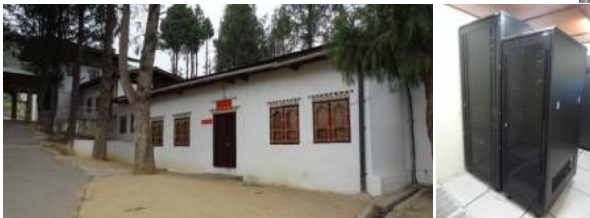
Figure 17. Health Help Center building (left); unanchored servers for the 112 emergency system (right)
