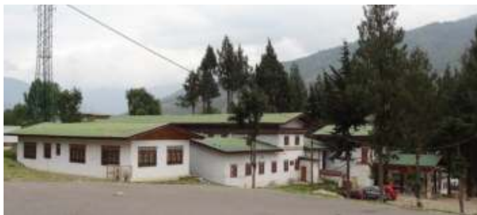
Figure 13. Overall view of main complex of community health buildings
