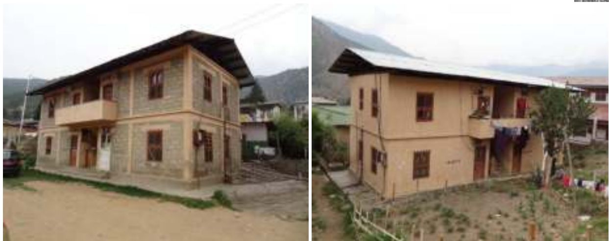
Figure 25. Nurses quarters (Type 1a) with 4 units built of concrete block with some concrete columns; unplastered (left) and plastered (right)
