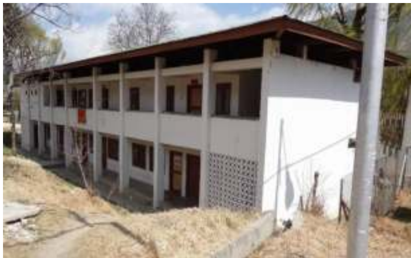
Figure 19. Maintenance office building
