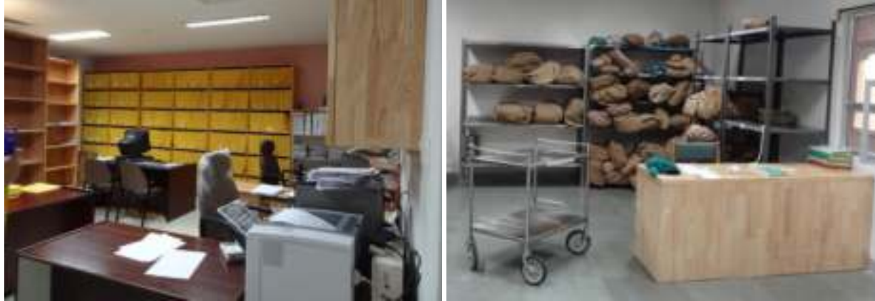
Figure 42. Large, unanchored medical records shelving (left) and unsecured racks in CSSD (right) near staff workstations
