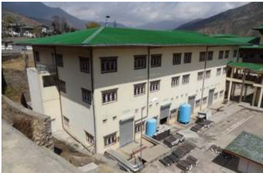
Figure 8. Exterior view of Service Block taken from top of retaining wall behind hospital, showing tanks for vacuum (blue) and empty medical gas cylinders awaiting pickup. Bridge to main hospital is at right.
