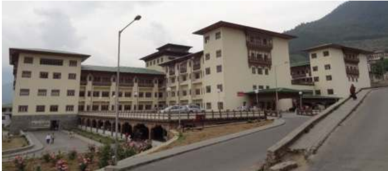
Figure 5. Exterior view of new Main Hospital Building showing parking garage (lower foreground), main entry (left) and ambulance entry for emergency department (right). Note captive columns (see page 20) caused by partial height masonry walls and decorative Zhu in parking garage.
