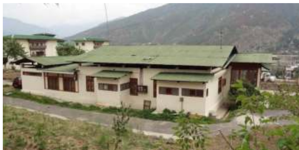
Figure 21. Medical Superintendent's quarters with the main hospital in the background
