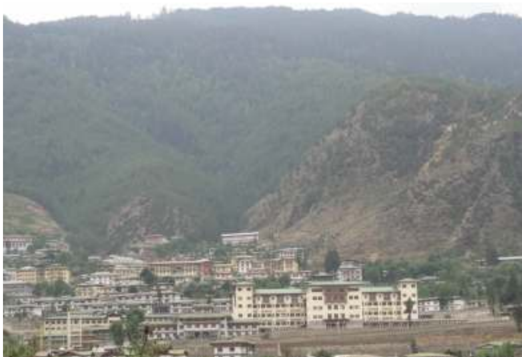
Figure 3. Topography near the hospital (pale yellow building in foreground); note large retaining wall in front of hospital
