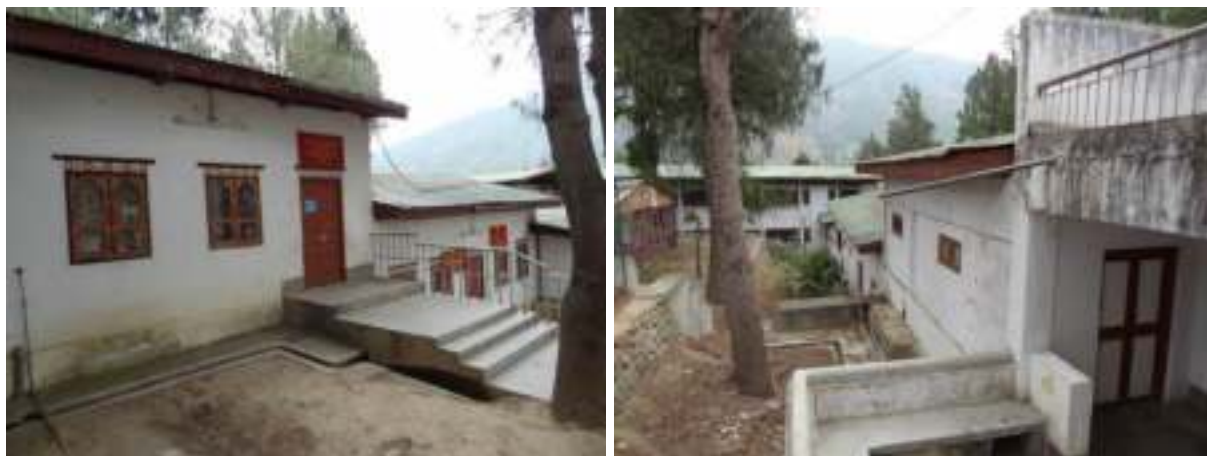
Figure 15. Front (left) and rear (right) views of Hand Therapy Clinic and TB Unit and Voluntary Testing Unit Building
