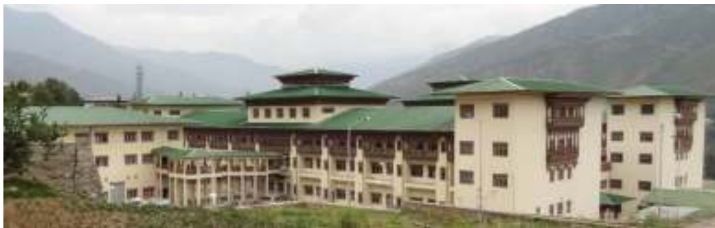
Figure 6. Rear view of Main Hospital building showing location of Service Block (at left) and connecting bridge (center)
