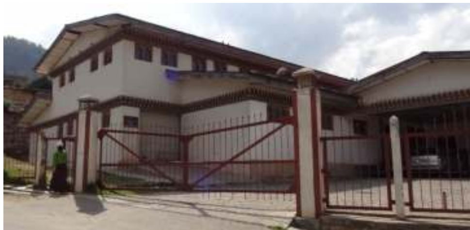
Figure 31. Portion of the DVED building complex housing the Central Medical Store
