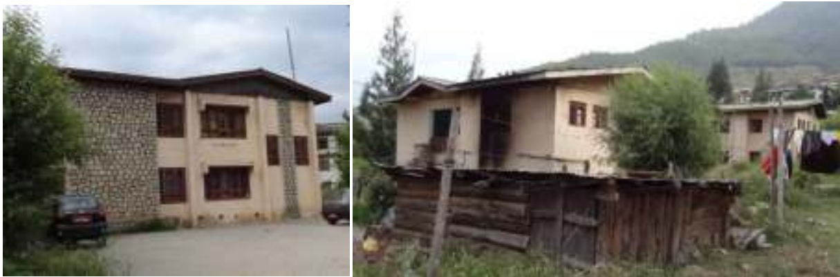
Figure 24. Multifamily doctors quarters
